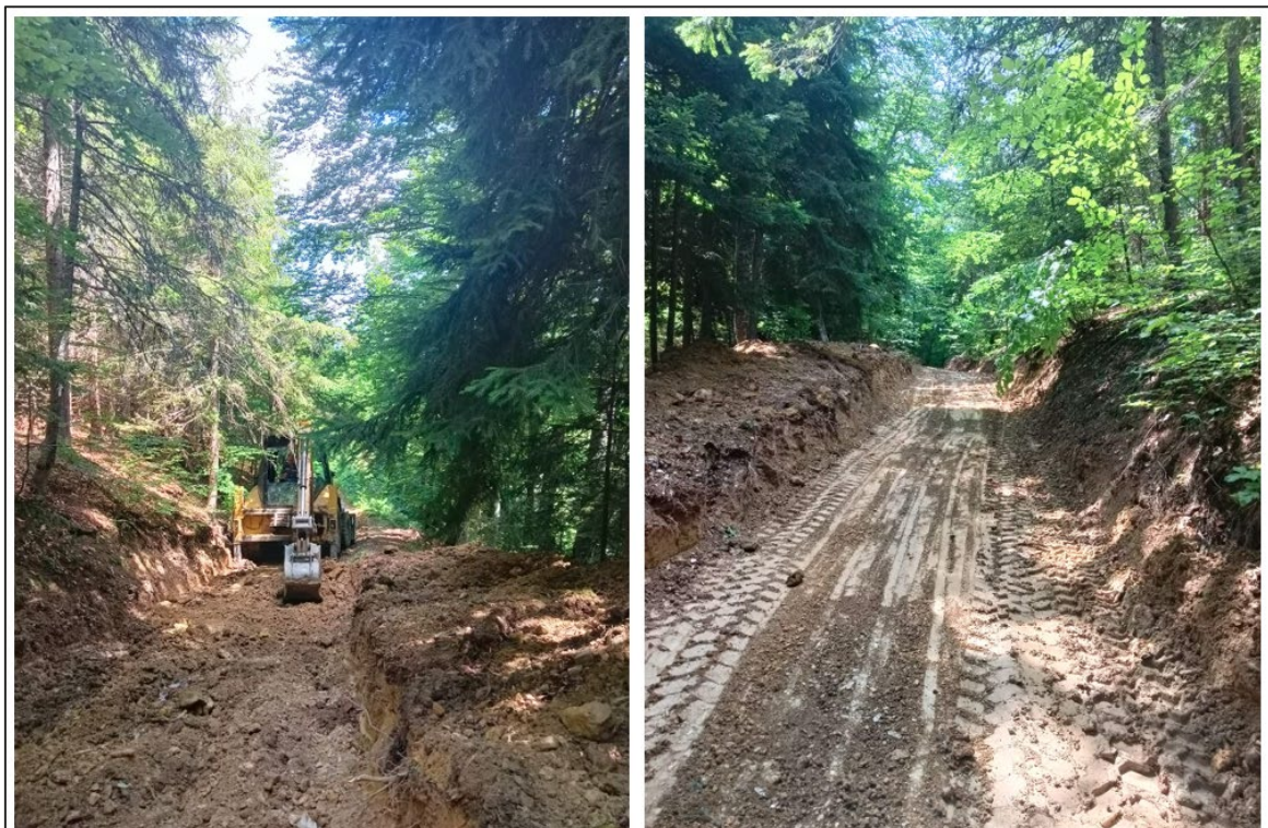
Figure 5: Monte Project, Pisonica Ag-Pb-Zn Prospect, photos of forest track repairs for drill site access
