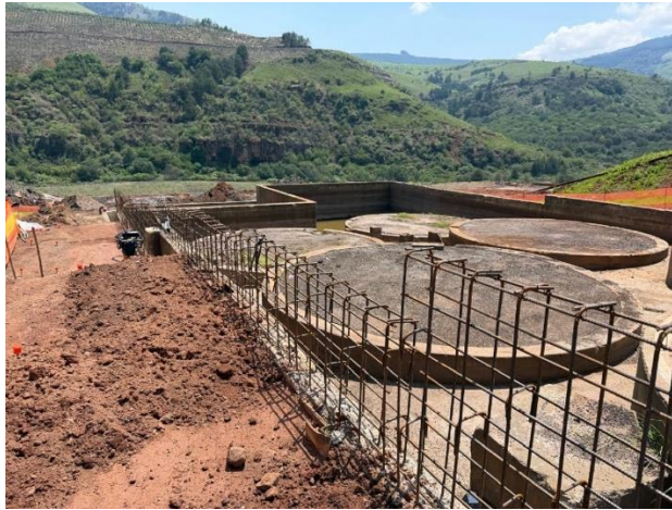
Figure 8: Steel reinforcing installation at CIL section
