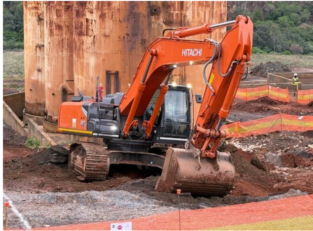
Figure 9: Excavation work for Gold Room
