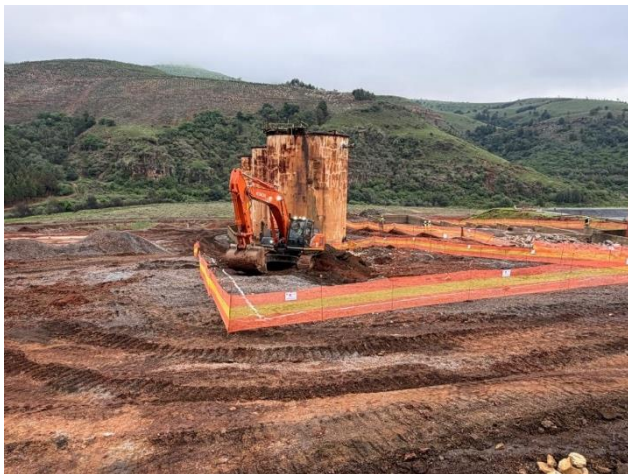
Figure 4: Earthworks for the gold room foundation works
