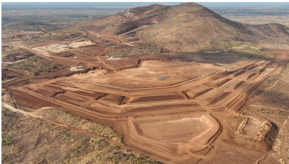
Picture 4. Tailings Storage Facility at Kangankunde
