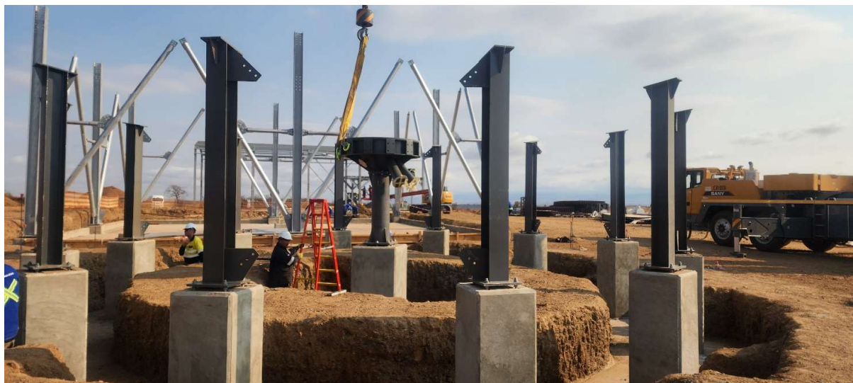
Picture 3. Thickener civils and structural installations
