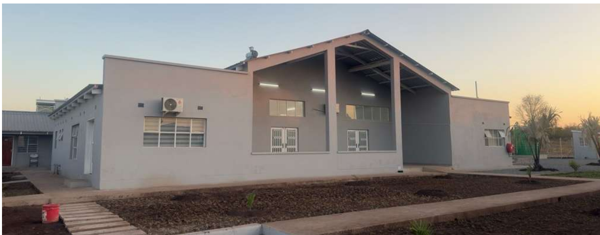
Picture 5. Operational mess facility at Tipume Accommodation Camp
