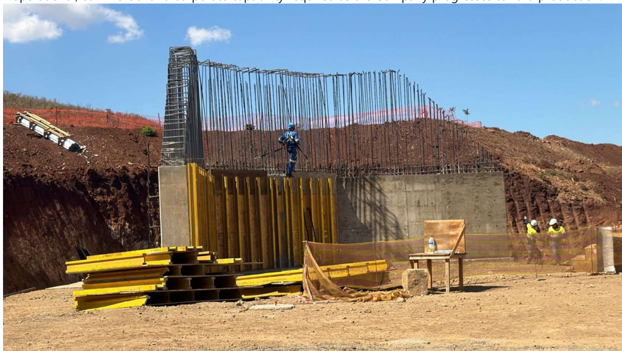
Picture 9. ROM pad civils advancing
