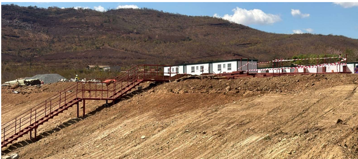
Picture 6. Phase 2 accommodation camp extension
