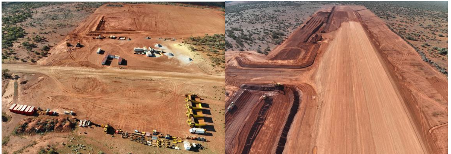
Figure 5 | Dingo Range Gold Project civil works, Left: Plant site Right: Airstrip
