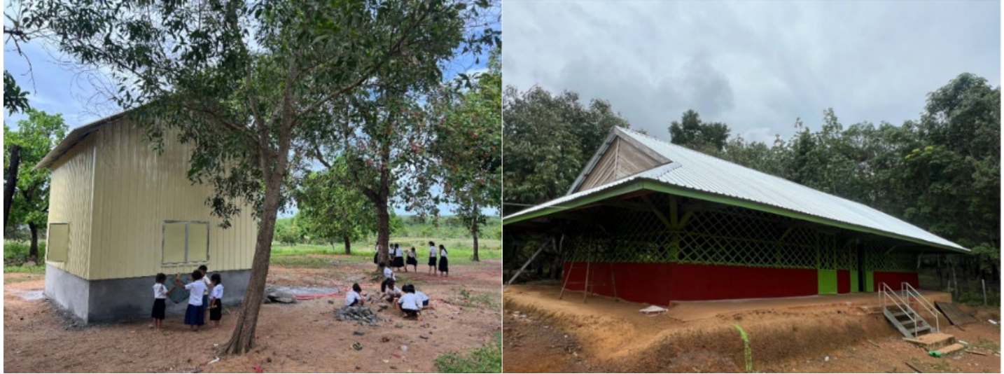
Figure 29 | Left: Don Pov Primary School New Library, Right: Kombas Primary School Roof Repair
